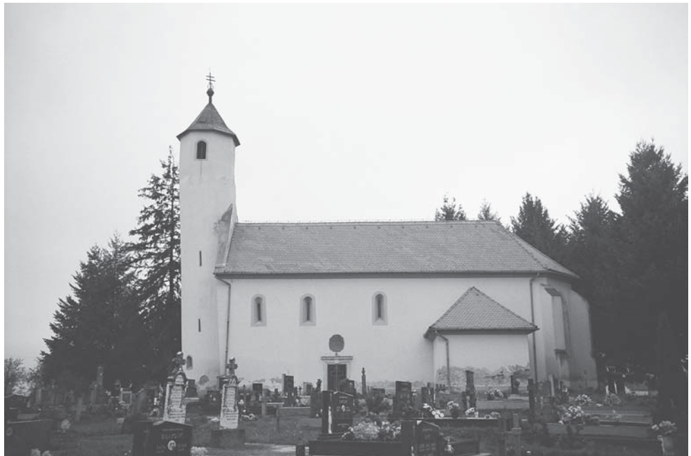
2. The church of St. Bartol at Novi Mikanovci, first half of the 13 th century. Photo: Archive of the author.
