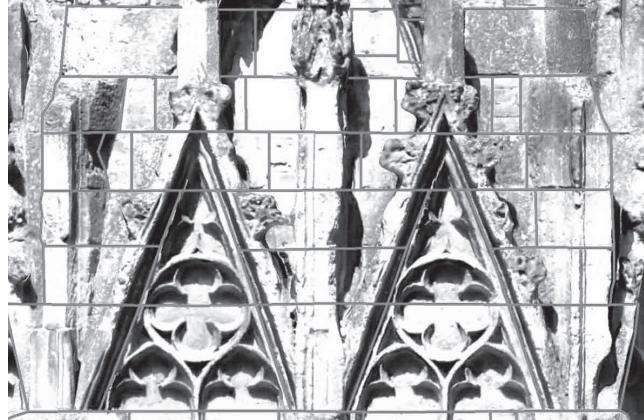
Fig. 8.: the joint structure of the gables on the reconstruction plan, the joint structure of the same part on the garden pavilion. Reconstruction plan: Gyula Forster National Centre for Cultural Heritage Management, orthophoto and joint structure of the garden pavilion: author
